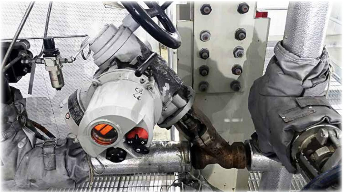
**The steam control installation before replacement of valves and controls. Original equipment had issues with leakage and damage to controls that impacted maintenance reliability. To make matters worse, there was no service support from the component manufacturers.**
