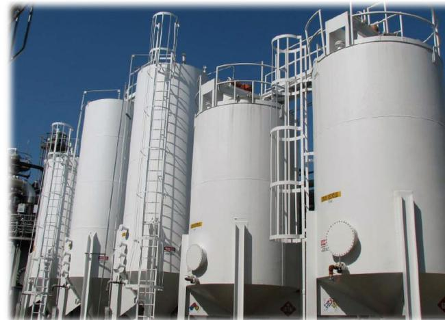
*The chemical production process burns molten sulfur to create sulfur dioxide which then is absorbed in towers converting it to ammonia bisulfite (ABS).*
