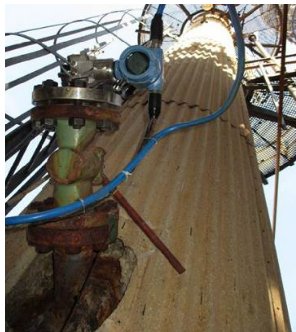
Rosemount 3051ERS installation
