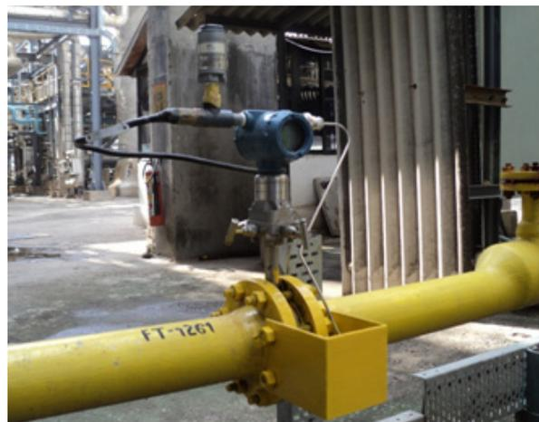
*Wireless gas flow measurement with Rosemount Conditioning Orifice Flow Meter and THUM was easily integrated into the plant DCS.*
