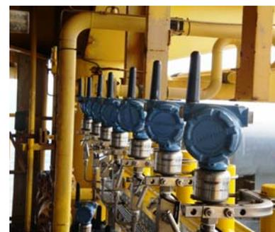
Casing pressure monitoring on 16 well-heads
