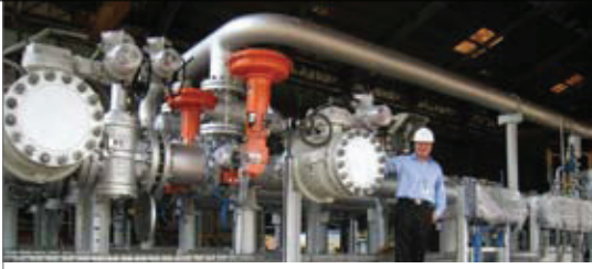
Figure 6: One of the 76 metering skids built for Reliance refinery in Jamnagar, India, the world's largest refinery. The metering systems were manufactured in Daniel's Singapore facility to monitor oil and gas valued at $27 billion.
