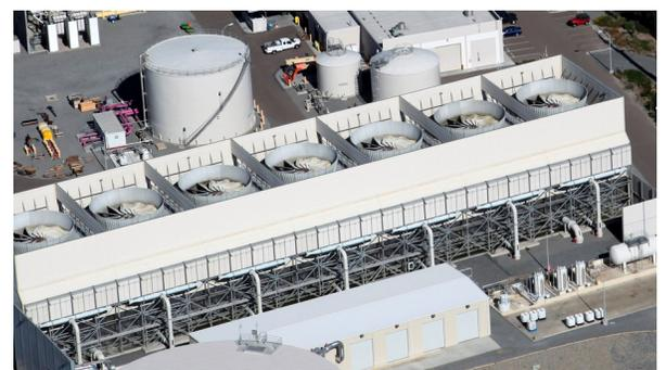
*Wireless now provides cooling tower riser temperatures which are used in the efficiency calculation to confirm the fans are running at correct speeds. This enabled the power plant to stop over-compensating, which has improved thermal efficiency.*
