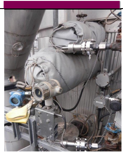
Rosemount 3051S Thermal Range Expander installation in application #1
