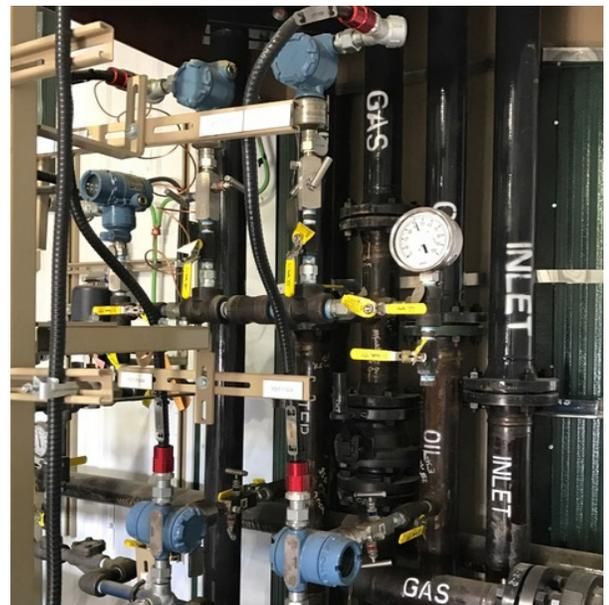
Rosemount 3051S ERS installed on oil leg.
